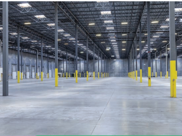
ESFR SPRINKLER SYSTEMS
